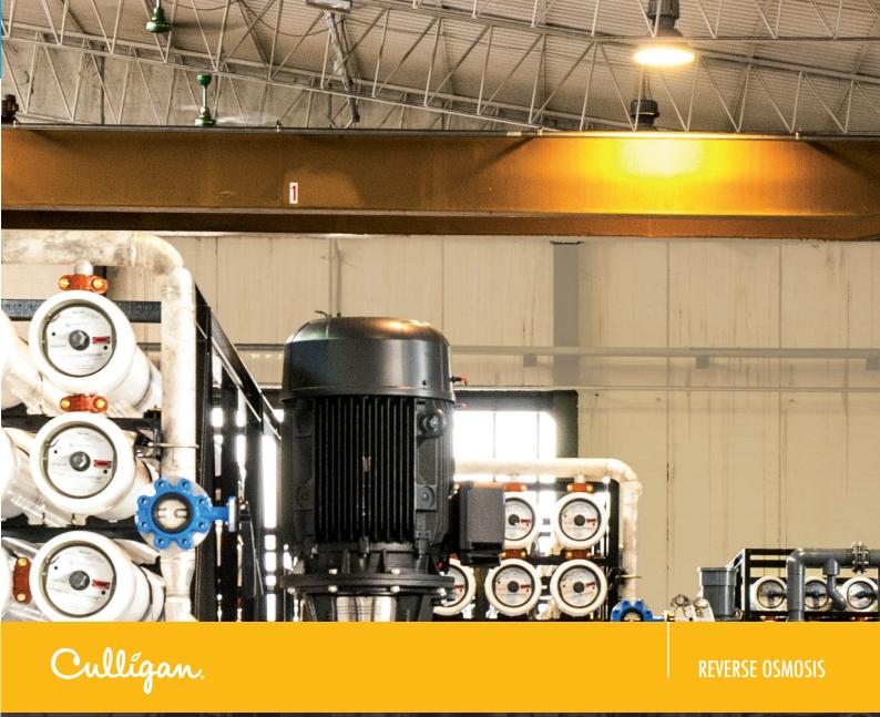
Reverse Osmosis (R.O.) exploits the ability of semi-permeable membranes to separate the water from the substances dissolved in it. Applying a pressure, the water is forced through the membrane: pure water (permeate) will thus be separated from the water containing salts (reject).
