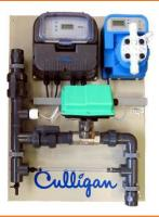
The Automatic Blowdown for Cooling Towers includes a management/programming controller, conductivity meter, conductivity cell with continuous reading, motorized valve, metering pump for shock biocide dosing, sampling point, electric and hydraulic interconnections between the parts.
